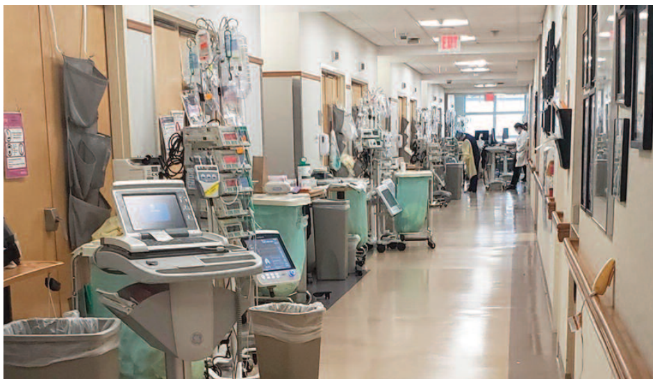
Figure 1. Pumps lined up outside patient rooms in a hospital ICU (March 2020).
